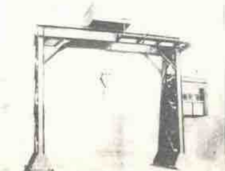
Traveling gantry crane as employed at transfer points of railroads where volume of freight to be transferred is too great to be economically done by a stationary gantry crane, as illustrated at the left.
