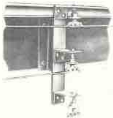
Bare copper wires stretched the length of the building and supported on insulators spaced at 20-foot intervals along runway. Bridge collectors raise wires off the insulators as crane passes. This system, known as "Shaw-Box" Type "Y" system.
