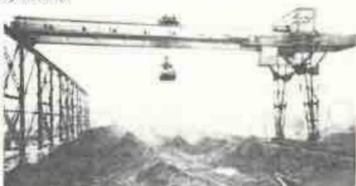
Single leg coal handling gantry crane employed to unload and rehandle all the coal used by a large power plant.
