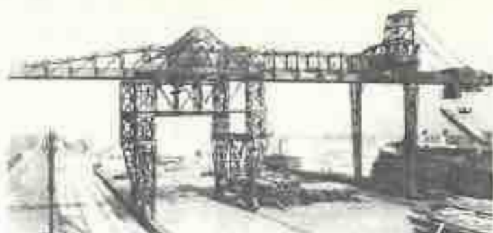
An unusual type of gantry crane. This crane is 200 feet in length and has a lift of 85 feet. It is used to unload miscellaneous material from ships, lifting it from the ship and depositing it on the platform shown on the left of the crane and then the entire load is transported along the dock by the crane.
